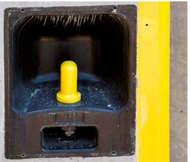
Recessed bollard for u- or Z-sections
