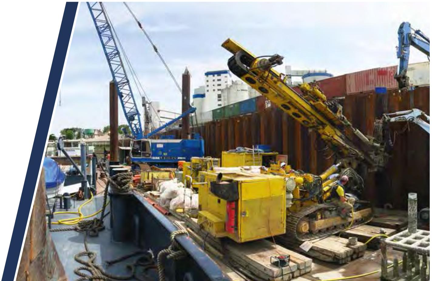
**TK-ASF grouted anchors, despite their small diameter, make use of special pressure grouting methods to transfer extremely high service loads into the subsoil.**
