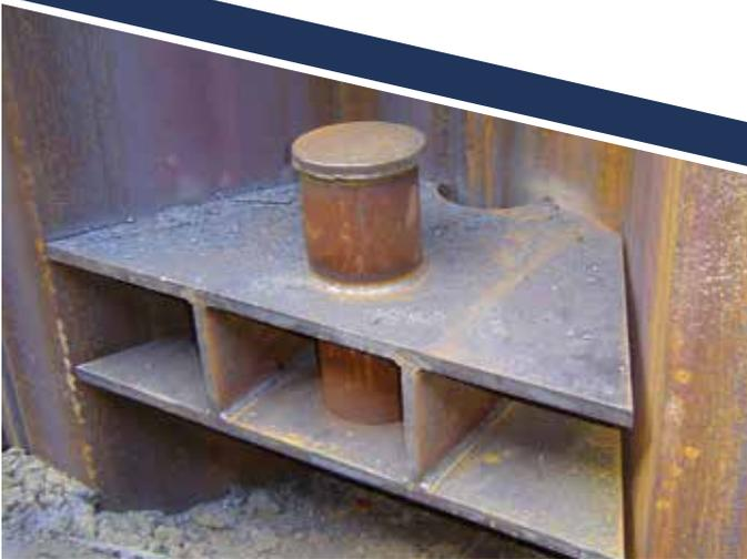
Break-off anchorages designed for the nominal load can be provided to avoid excessive line pull loads from overloading the sheet pile wall.
