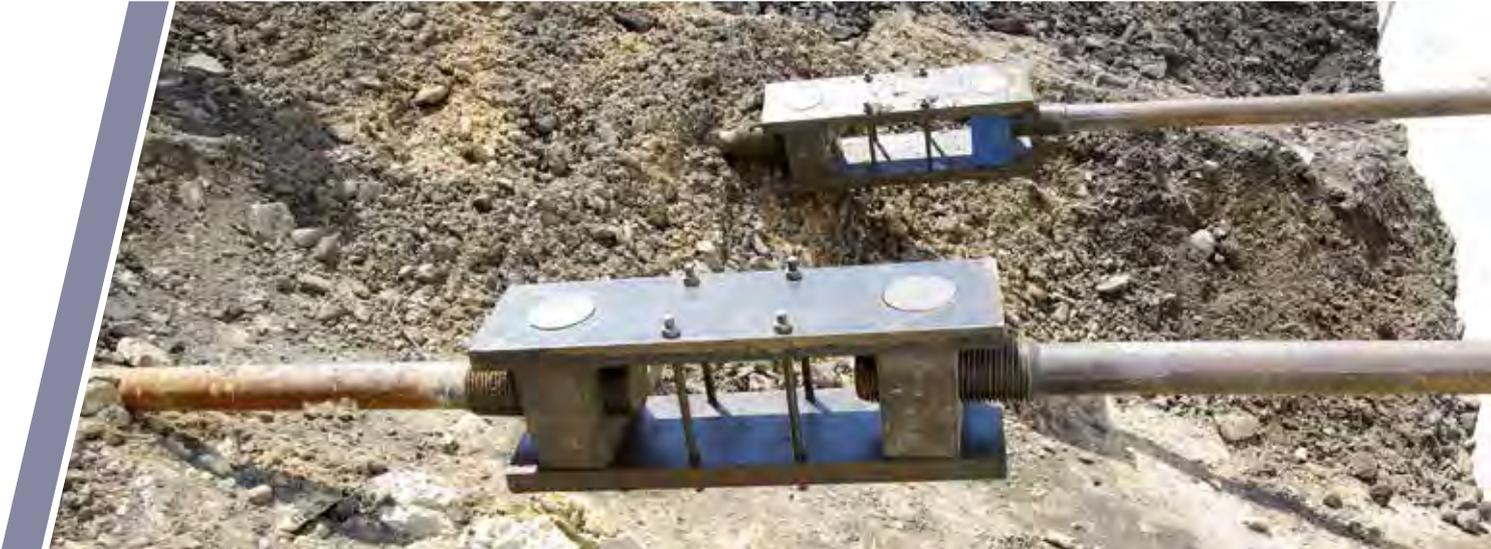
Turnbuckles have left- and right-hand threads for tensioning the anchorage and adjusting the total length of the anchor.
