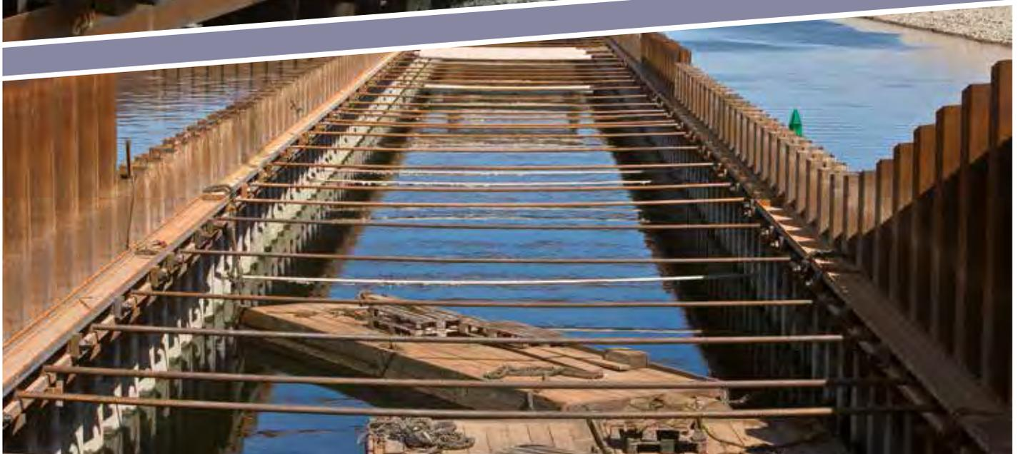
If the structural and constructional requirements placed on a sheet pile wall call for an anchorage, then propping the walls against each other is one way of doing this, e.g. in trenches for installing buried services.
